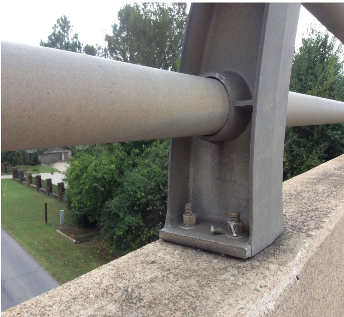
PHOTO 1 Description Loose bridge rail. Connection bolt laying on the base of the post.
