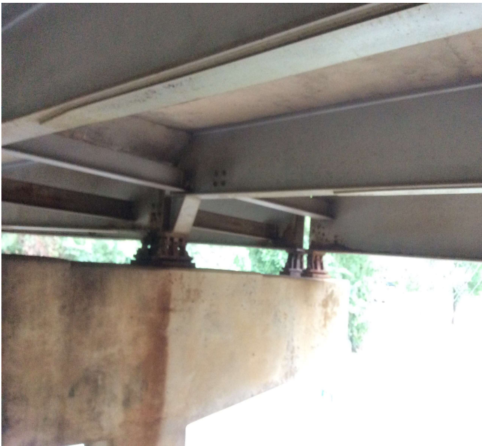
PHOTO 3 Description Bent 3 Beams 1&2 corrosion
